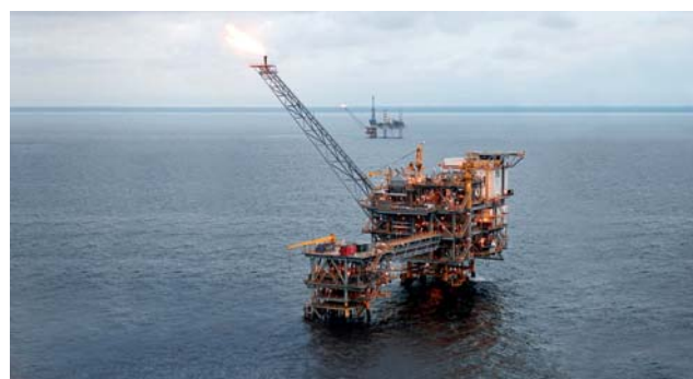
Okume Complex production platform, offshore Equatorial Guinea.
